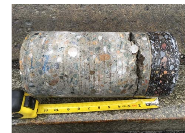
Bridge deck core, determining the location of the rebar meshes
