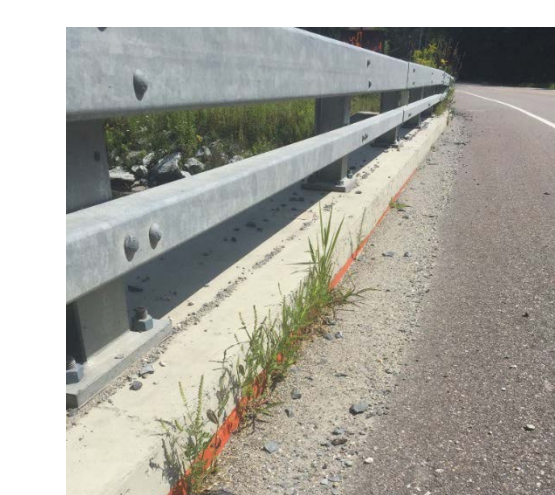
Close-up of Bridge 165 bridge deck showing evidence of BDM system
