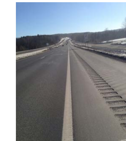
Pavement marking liquid paint study on I-89 between Brookfield and Montpelier
