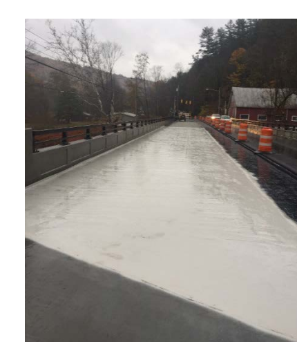
Eliminator membrane installation, Bridge 11R on VT 121 in Saxton's River
