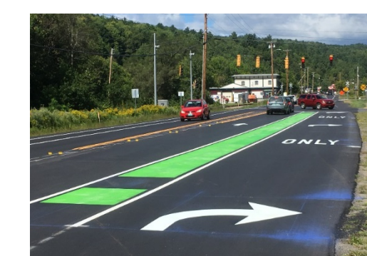
Pavement marking tape study (long lines, symbols and bike lanes) in Berlin
