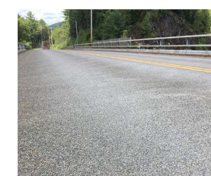
Poly-Carb Flexogrid, Bridge 8 over I-93 in Waterford
